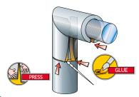
4 Sheath the elbow joint with the sleeve and glue the cut edges together, press to bond and continue cladding with straight sections of TROCELLEN sleeve of the same diameter
