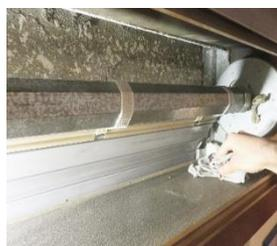
**1. Disassemble the removable side of the box and make a first inspection** with the aim of detecting its conditions, **removing dirt, dust, and any residual of other materials**. The internal surfaces of the box must be clean to facilitate installation of self-adhesive band.
