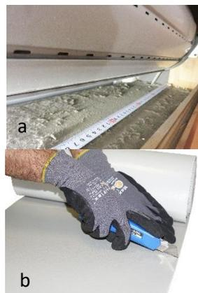
**2. Take measurements** of the surfaces to be insulated (front panel, sides, back and bottom) **(a)**, as well as the thickness available for the insulating material (thickness between roller shutter, when completely inside the box, and the panel itself). **Cut to size** the insulating material **(b)**.
